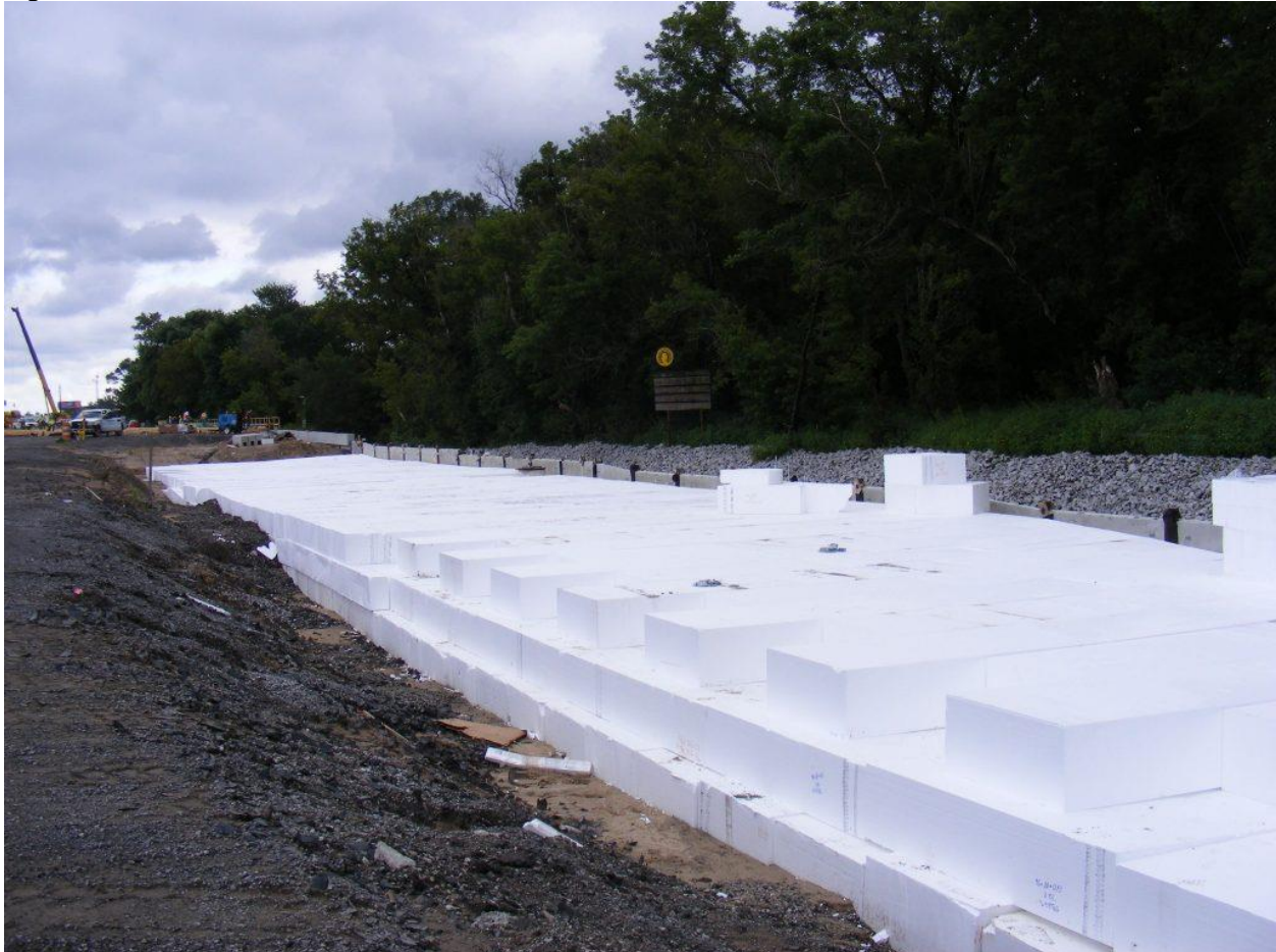
Figure 10: EPS Foam Fill
